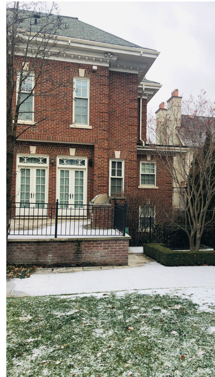
EXISTING BACK FACADE & YARD
