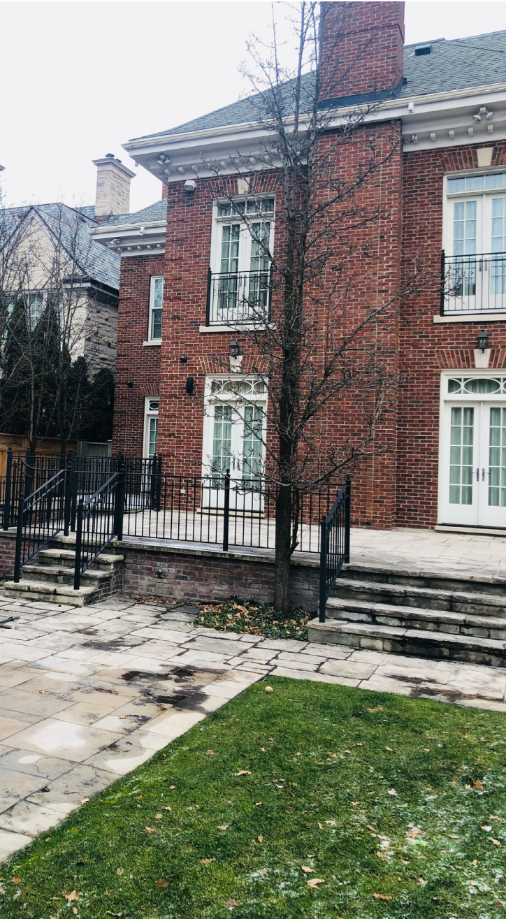
EXISTING BACK FACADE & YARD
