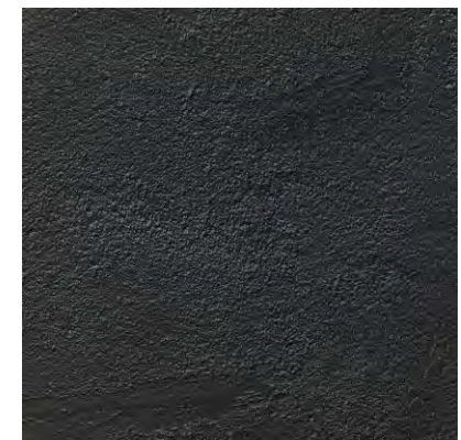
BLACK PLASTER WALLS
