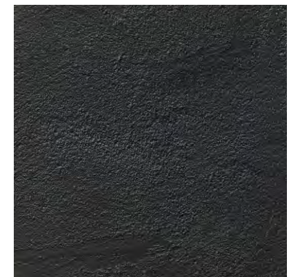
BLACK PLASTER WALLS
