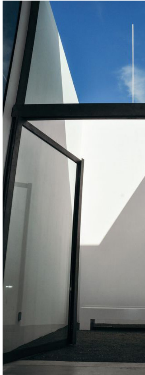
FULL HEIGHT GLAZING
