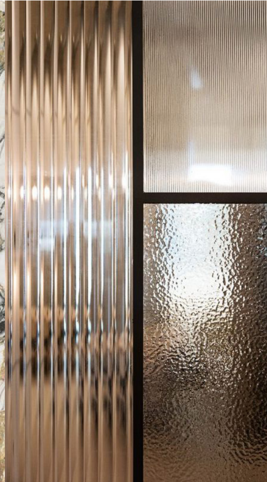
FROSTED AND REEDED GLASS ON DOORS
