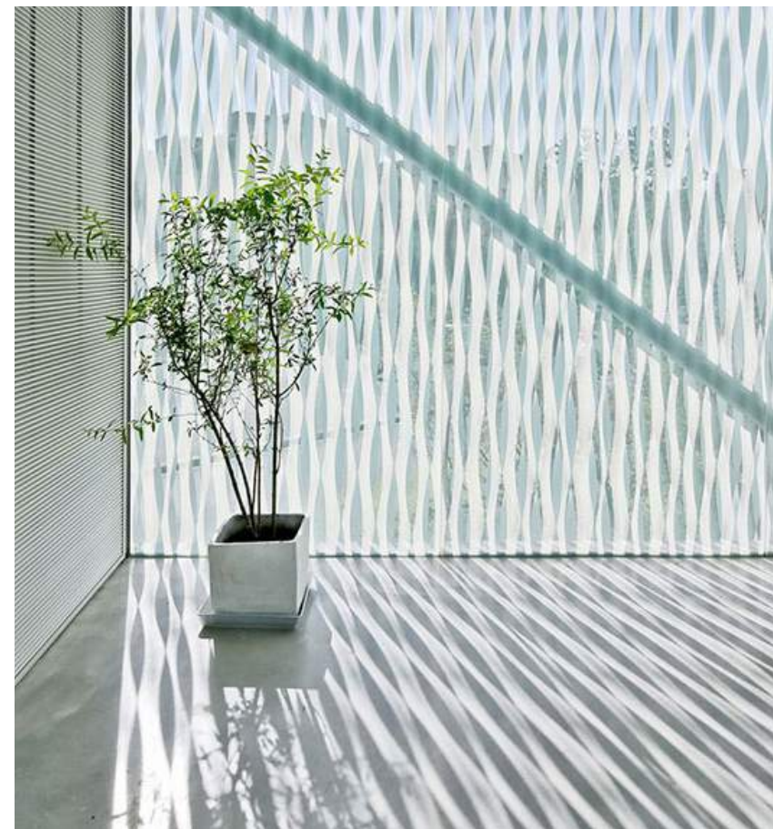
FRITTED GLAZING TO VISUALLY PROTECT GUESTS FROM THE EXTERIOR VIEW
